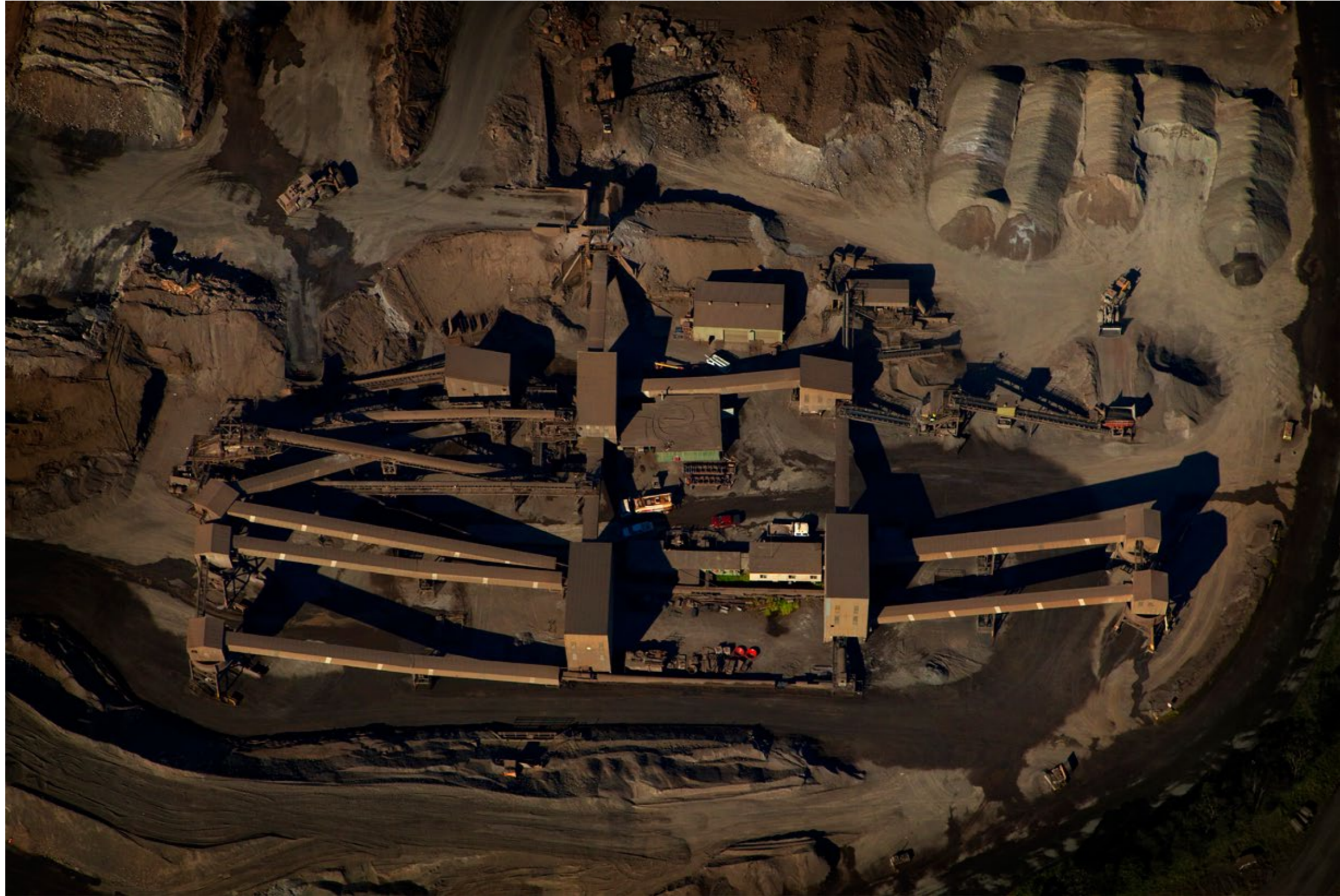
Recycling plant, Port Kembla, NSW, Australia. Canon EOS 1D MkII with 24-105mm L lens. © Geoff Comfort
